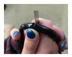
It will be easier to strip off sheathing before the tail is attached to the panel. Measure the distance from the attachment point to the furthest point and strip this length of sheathing from the tail. This can be done by gently scoring with a sharp Stanley or craft type knife around the sheathing and then bending the tail. This should open the score line and the sheathing will then pull off. Take care to not cut through the sheathing and score the fibres.
